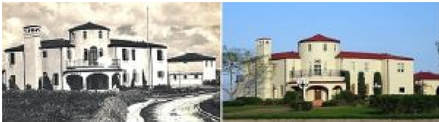
Donigan Home in 1933 and following renovation
